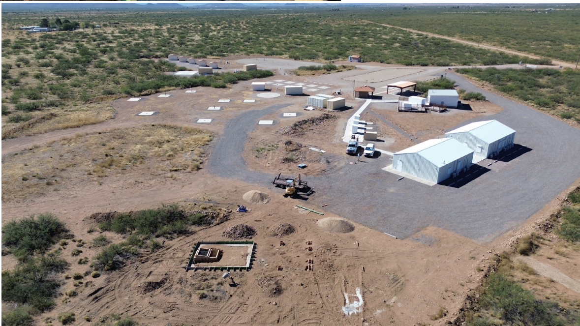
Foundation from east looking over site
