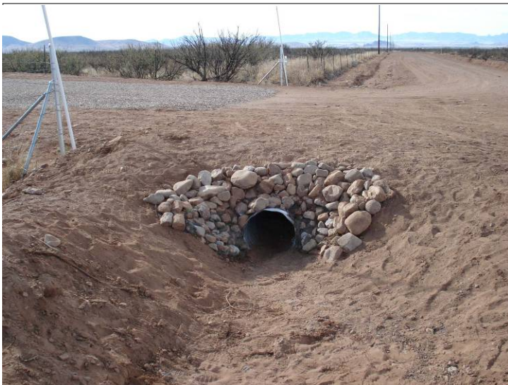
Culvert erosion protection
