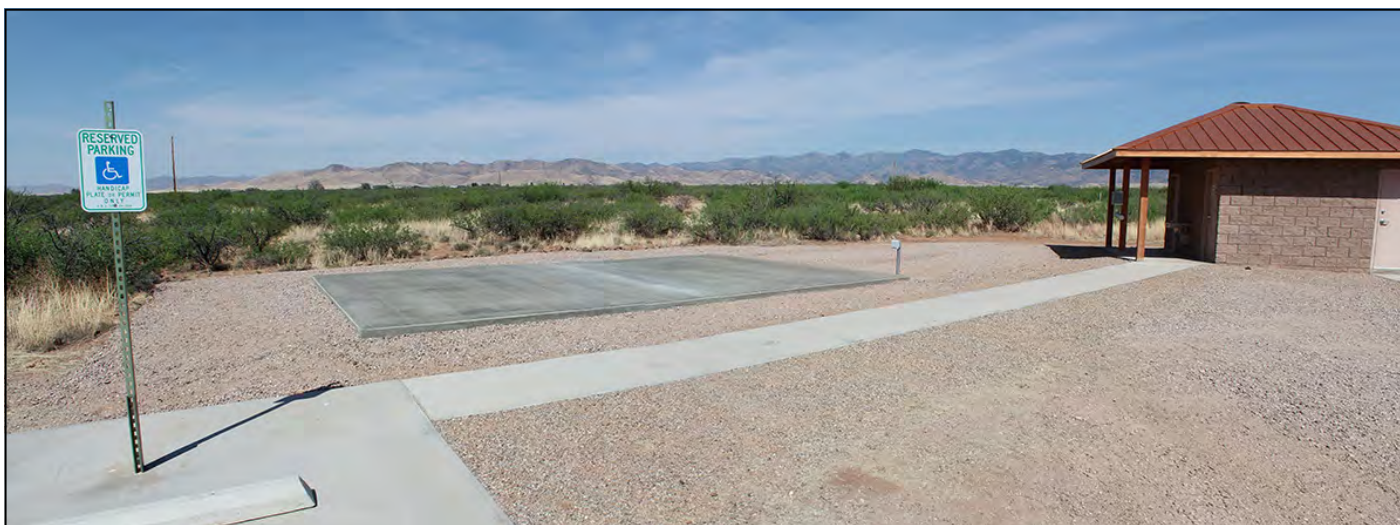
Concrete slab, measuring 20' x 30', will become a covered picnic ramada.
