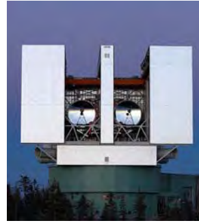
The Large Binocular Telescope. The top structure of the building (the white part) co-rotates with the telescope. Image by Mt Graham International Observatory.
