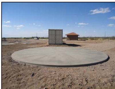
Amphitheater pad with storage container
