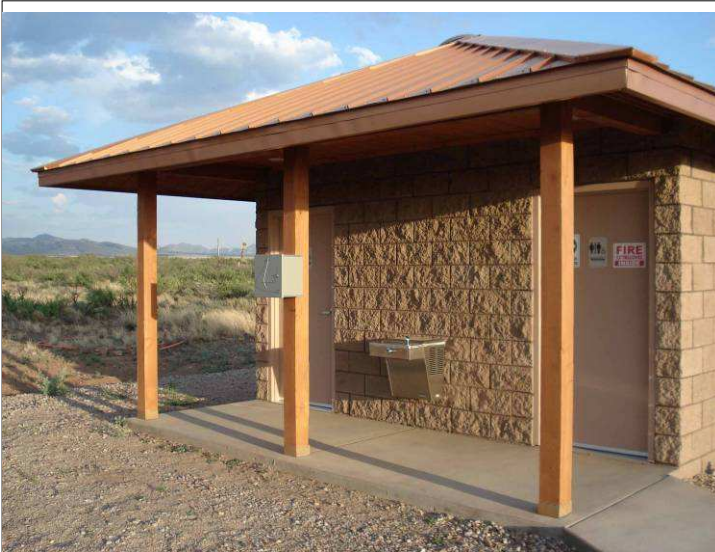
Key Safe Enclosure mounted at Bathroom Facility
