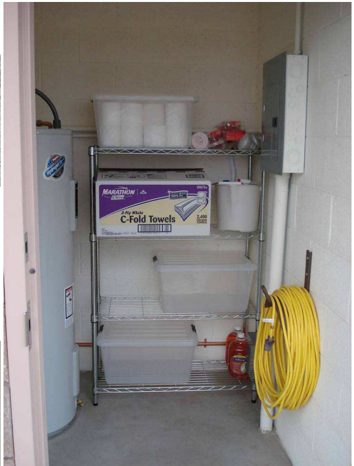
Utility room with storage shelves & supplies
