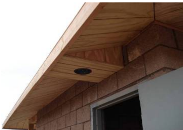
Bathroom Facility – Soffit paneling & light box installed
