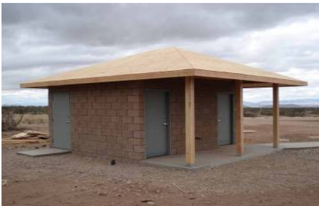
Bathroom Facility – Doors installed
