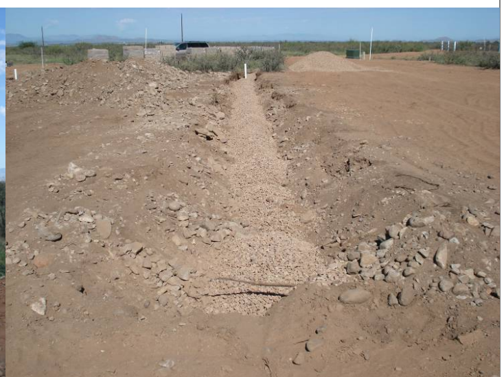
One Septic Leach Line Trench Awaiting Pipe
