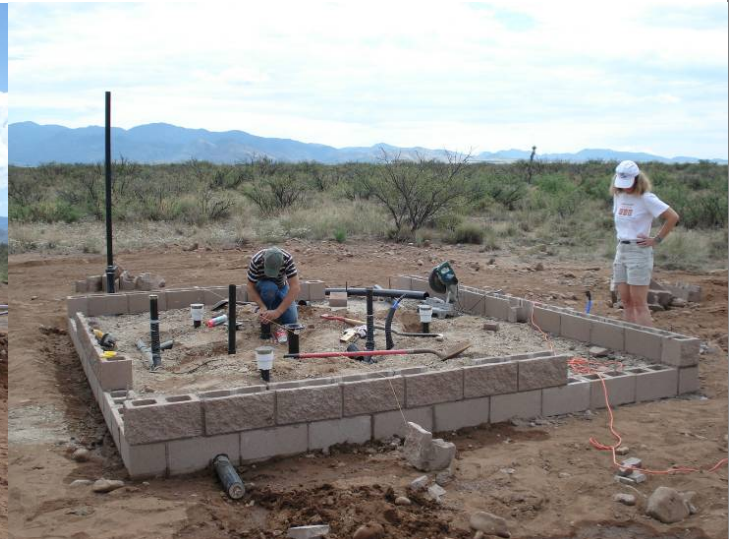
Bathroom Facility Sub-Slab Plumbing with Stem Wall
