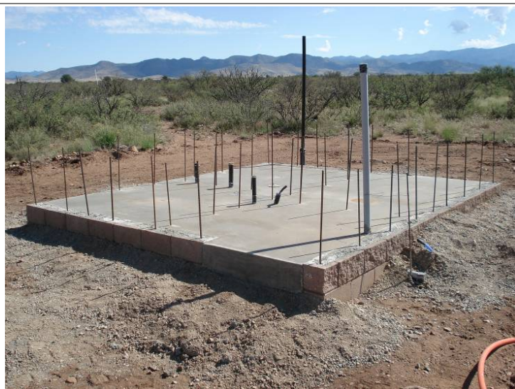
Bathroom Facility Finished Floor Slab
