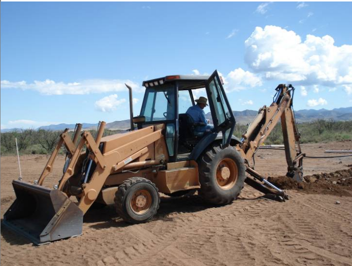
Peter Ammon Trenching the Septic Line
