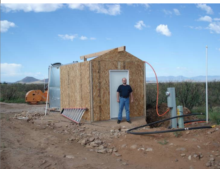
Preliminary Well House Construction
