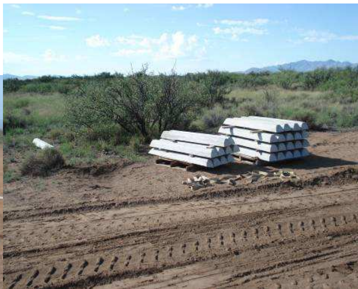
Concrete Parking Space Bumpers Delivered
