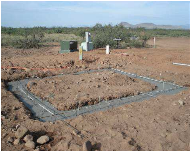
Bathroom Facility Reinforced Footer Installation
