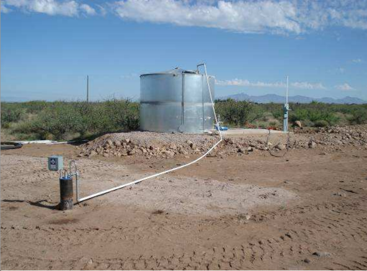
Temporary Well Set-up
