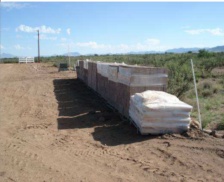
Bathroom Facility Concrete Blocks & Mortar Delivered
