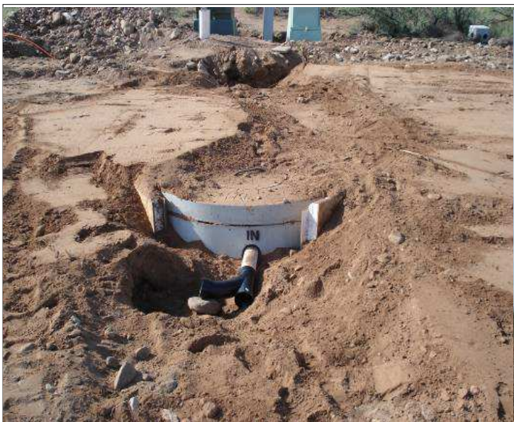
Septic Tank Installed
