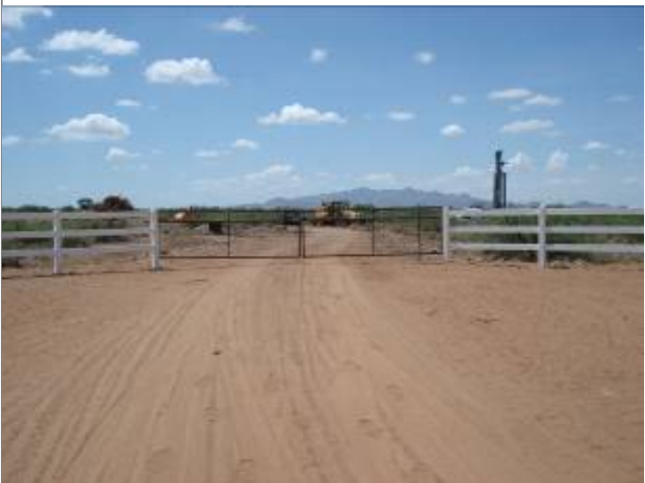
Entry road decorative fencing and gates.
