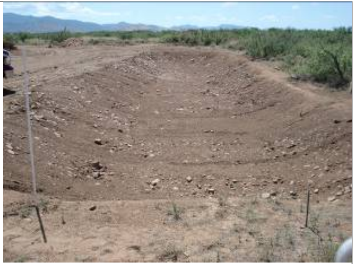
Rain water catchment "ditch" (will be lined with stone).
