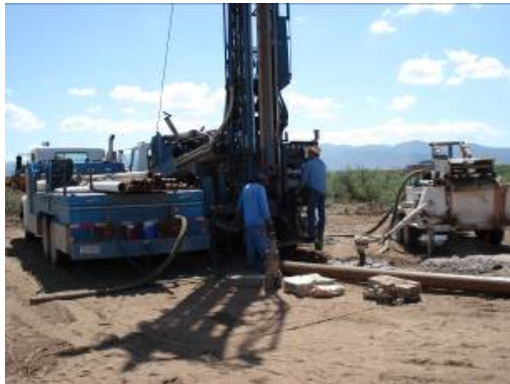
Well drilling operation.
