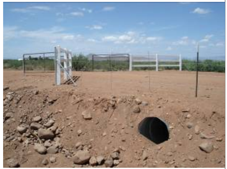
30" diameter culvert under entry road.
