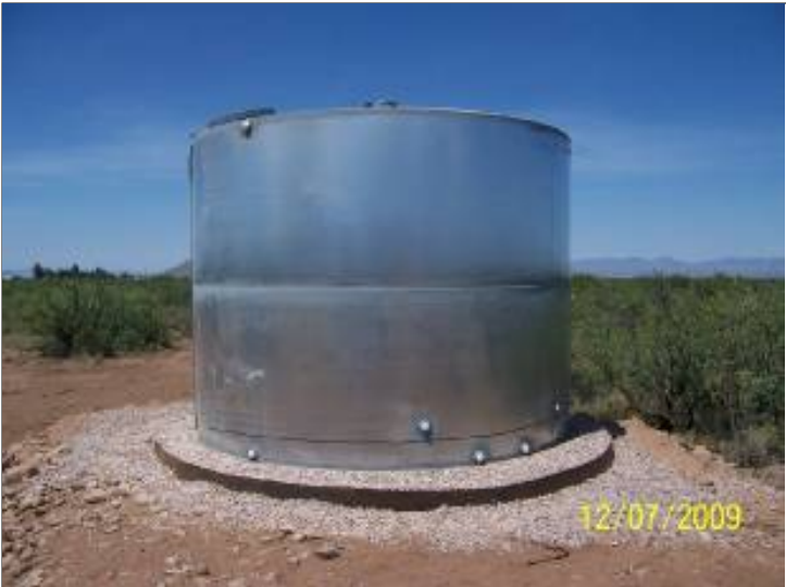
Five-thousand gallon water storage tank at well site.
